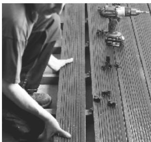
The Govadeck decking boards are always produced at a length of 360 cm. Small tolerances in the length are normal. The cross ends of the boards display extrusion rests. These need to be sawn off prior to installation.
