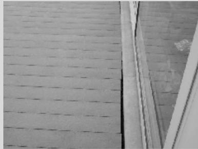
The bearing structure needs to be fixed onto the ground in one straight line to enable a controlled expansion. If it is not fixed, the structure may move slowly, as demonstrated in this picture.
