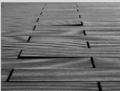
Although the boards are well installed in a staggered formation, they were not connected lengthwise and no double supporting beams were used. As a result, the boards have pushed up and joints are visible.
