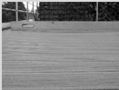
The boards are not sufficiently supported and there is too much space left between the supporting beams. This results in a floor area that has sagged.
