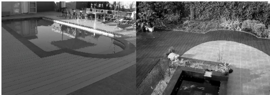
Two examples of decking installed finishing level with the surrounding ground. (No finishing border required.)
