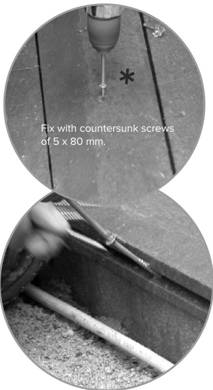
The fixation can also be done with invisible screws (see picture).
