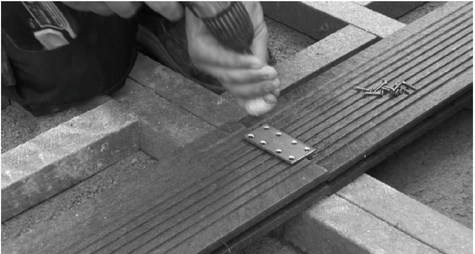
Connecting the boards lengthwise, will not only avoid an expansion gap between the boards, but also prevent them from getting pushed upwards where they are connected.
