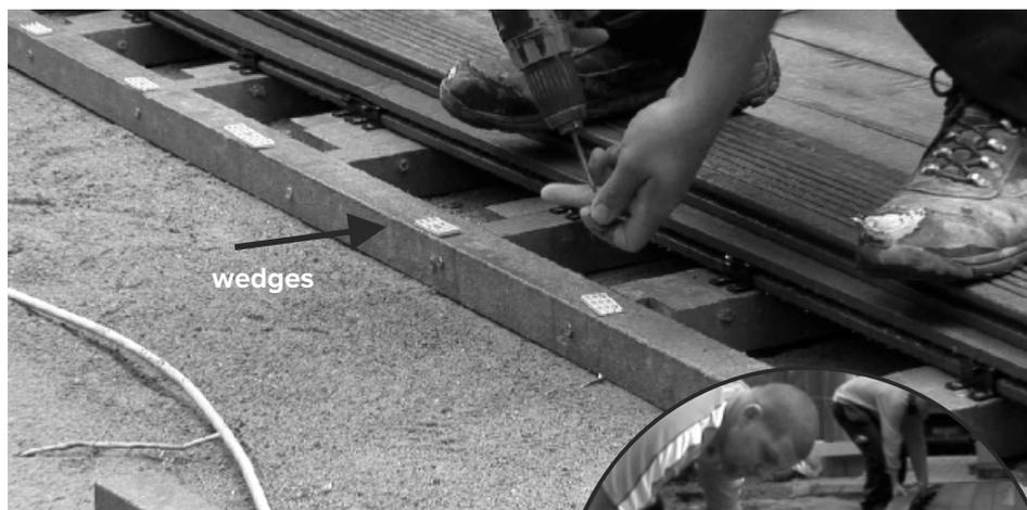
For the last board, no Gova-Connects are used, to avoid that the installation of the finishing board is obstructed. As an alternative for the Gova-Connects, wedges are used to fill the 3 mm space between the eco-beam and the decking board. The fixing of the last board is done with invisible countersunk screws of 5 x 80 mm, at the top or through the side groove (see picture).
