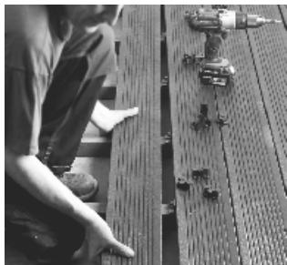
The Govadeck decking boards are always produced at a length of 360 cm. Small tolerances in the length are normal. The cross ends of the boards display extrusion rests. These need to be sawn off prior to installation.
