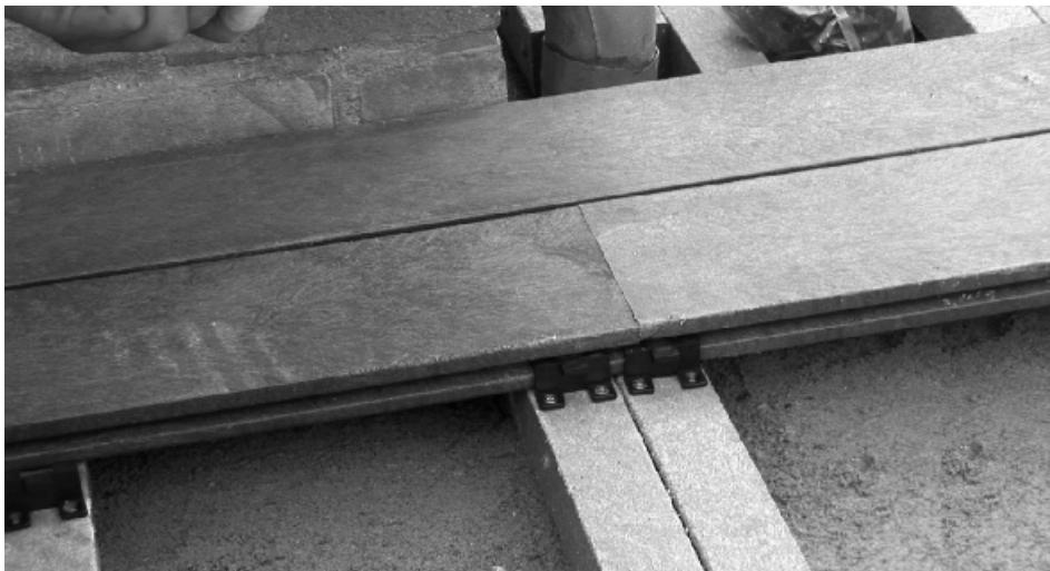
First the connection of 2 decking boards lengthwise is done with a Gova-Fix connection plate. Then the 'extended' board can be turned and put into the Gova-Connects.
