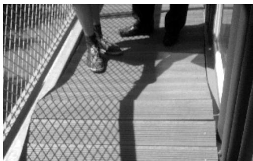
This picture shows the results of not properly taking into account the expansion of the bearing structure. These boards were installed during summertime, without the correct space being left to allow for the heat expansion effect; resulting in the distortion of the boards.
