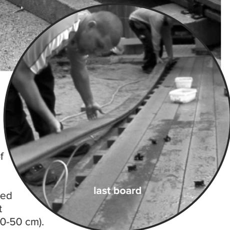
If desired, the deck can be finished with a border. With this method you can hide the bearing structure and the cross ends of the decking boards to obtain an attractive professional finish. The border can be the same colour as the decking board or alternatively another colour from the Govadeck® range.
